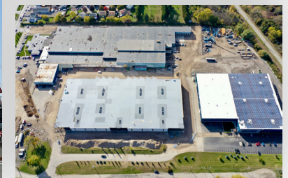
Left: Precast In-Progress Right Upper: Precast Complete Right Lower: Site Plan Aerial View
